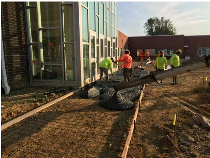
SVHS – Concrete sidewalk pour at front entrance.
