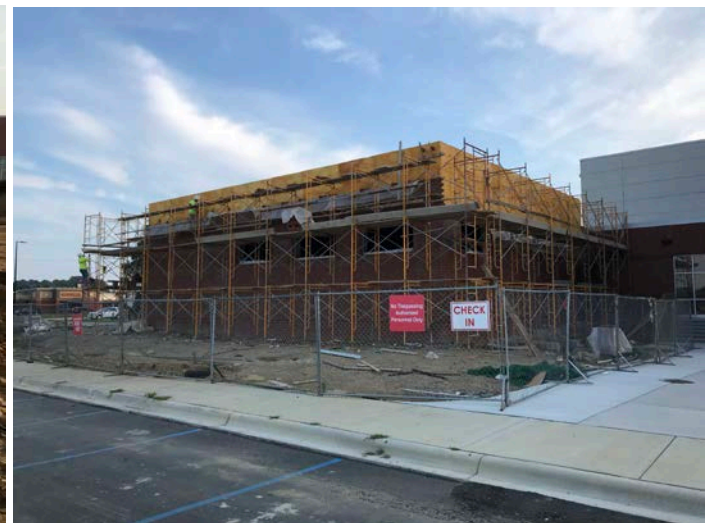
Construction of the weightroom building adjacent to the gym.
