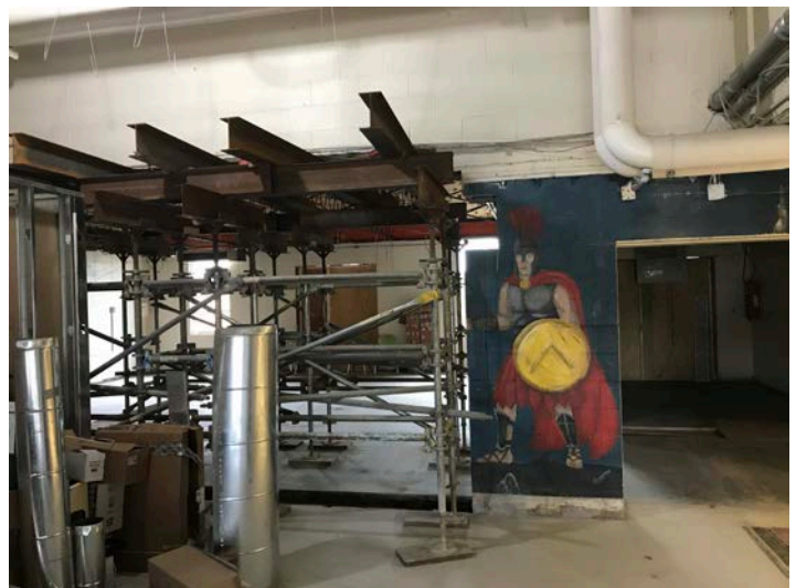
Temporary shoring for a new opening in existing corridor wall.
