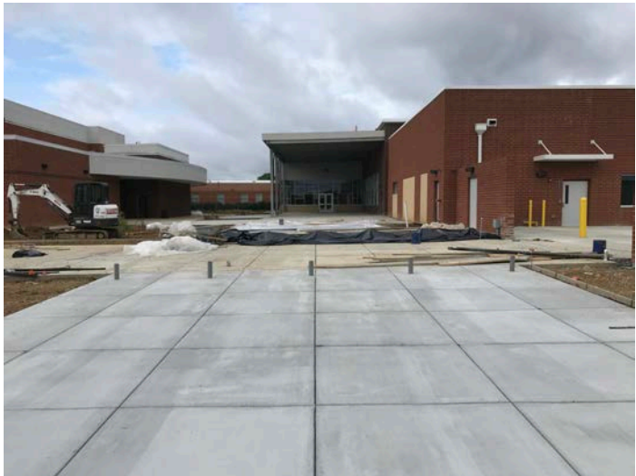
SVHS: Connecting concrete from school to stadium.
