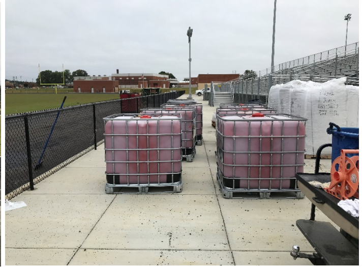
Final surfacing material for the track.
