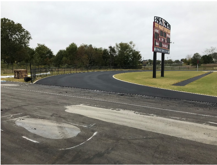
SVHS: Track synthetic surfacing underway.
